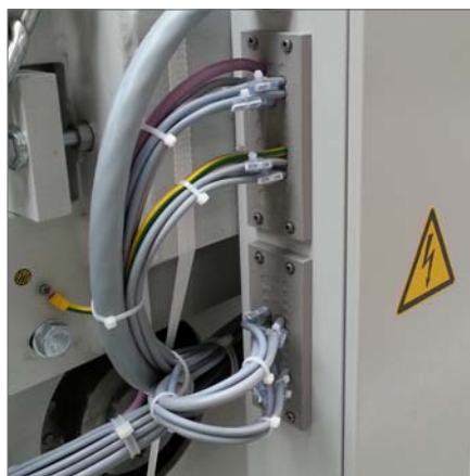
KEL-DPZ 24|x - Page 62 - 63 Routing of numerous cables with varying cable diameter sizes into a machine control panel. IP65 sealing is achieved. Additional membranes are available for future routing.
