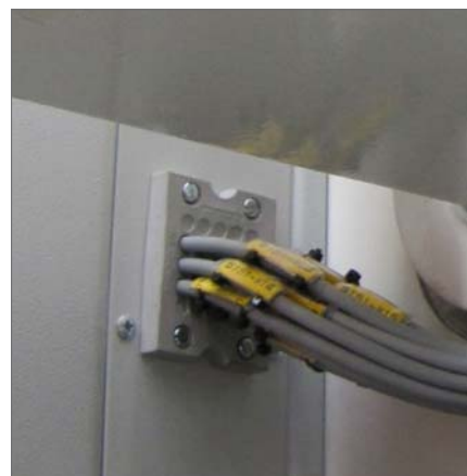
KEL-DPZ B25 - Page 64 Entering of cable bundle in a small space with high sealing rate IP66.
